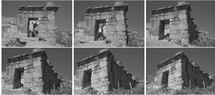
Figure 9.13: Image sequence which was used to build a 3D model of the corner of the Roman baths
